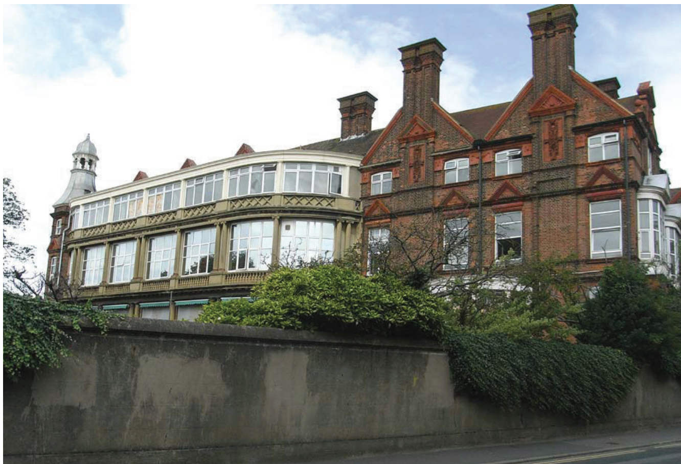
Former Royal Alex Hospital (Principal building)
