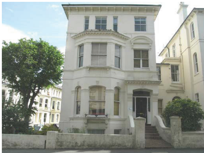
View of Dyke Road area
